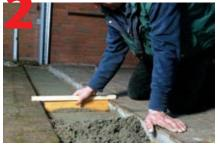
Lay 4" deep concrete bed. Cut channels to fit required length (if necessary).
