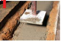
Excavate area to accommodate trench drain and 4" concrete surround, compact base.
