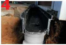
Push-fit outlet adaptor into bottom of channel, lay outlet channel first and connect to 3" or 4" SDR pipe or 4" schedule 40. Alternatively, use 4" flex coupling to connect 4" SDR pipe to outlet on base of corner unit, set in place and lay channels from that point.
